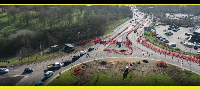
This scheme for Bedford Borough Council was a major junction improvement including a layout change to the junction, with associated signals works, road widening, drainage system and gully works, street lighting, service diversions, and civils on one of the busiest access routes to Bedford, whilst maintaining flow of traffic into and out of the city.
