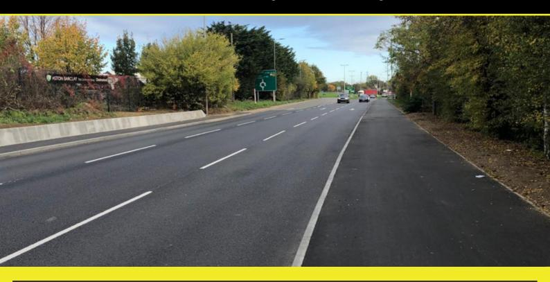
Running from July 2018 to September 2019, the project saw the widening of existing colchester road to create an additional traffic lane and a combined cycleway/footway. This required widening construction, realignment of drainage, new street lighting, installation of a new signalised pedestrian crossing, numerous sevice diversions and protection works, full resurfacing of the carriageway, and all associated road marking and traffic signs.
