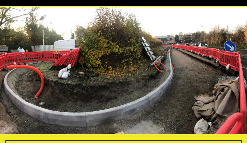
The Lawn Lane/Channels project saw Henderson & Taylor creating an additional lane to ease traffic flow at the junction of Rectory Road with Chelmer Valley Road. The project involved planing out, embankment stabilisation, drainage, kerbing, utilities management, and surfacing, as well as building a tobermore retaining wall to widen the road without disturbing the adjacent cemetary.
