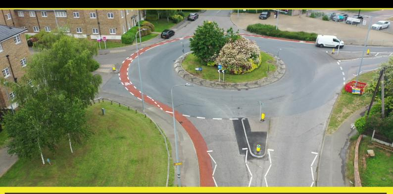
To improve safety and encourage active travel on around the school on Panfield Road, Braintree, Essex Highways contracted H&T to install a new cycle lane in distinctive red tarmac to give a clear route for cyclisgt along the road and around the roundabout.
