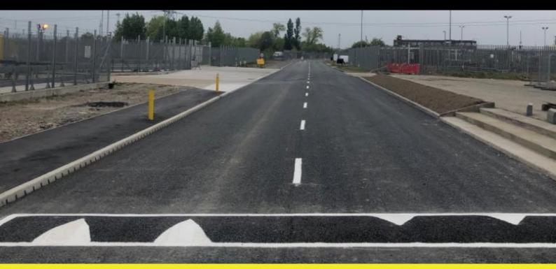
Restabilising the access road into the Corringham Refinery involved excavating and removing flooded area soft spots before replacing them with rock-fill, overlaid with a reinforced concrete raft, with a final surface layer of asphalt, as well as all lining, signage, landscaping, and associated drainage works.
