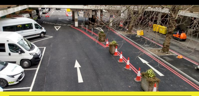
The project at Guy's & St Thomas Hospital saw H&T constructing and redeveloping the highway network for a busy central London hospital. Over a 15 week period we completed DDA walkways, deep drainage, surface elevation, associated kerb works, paving, and surfacing.
