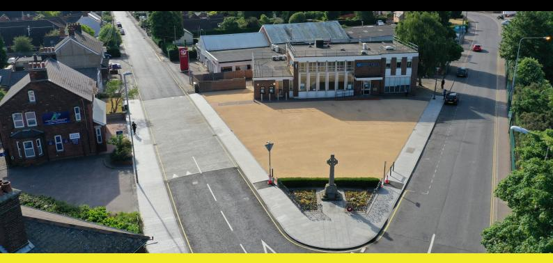
The Flitwick Town Centre regeneration project consisted of site clearance, resurfacing of existing roadways, new kerbing, new stone paving to footways, drainage works, a tactile paving crossing, resin bound surfacing, and all associated lining, signage and street furniture.
