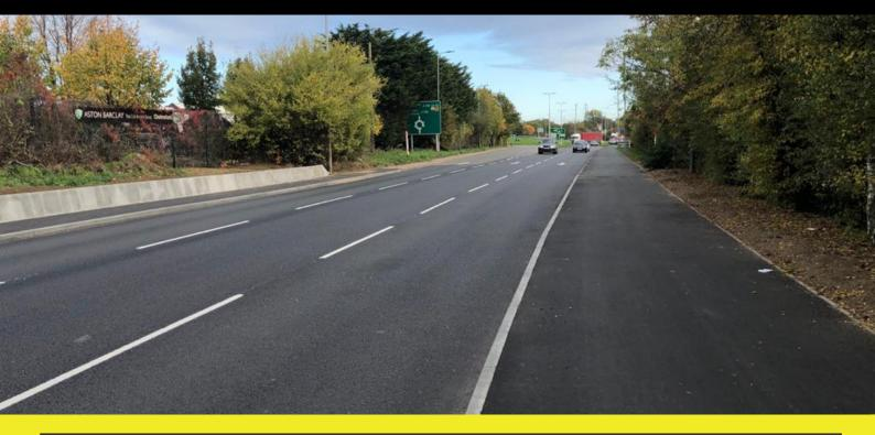
Running from July 2018 to September 2019, the project saw the widening of existing colchester road to create an additional traffic lane and a combined cycleway/footway. This required widening construction, realignment of drainage, new street lighting, installation of a new signalised pedestrian crossing, numerous sevice diversions and protection works, full resurfacing of the carriageway, and all associated road marking and traffic signs.
