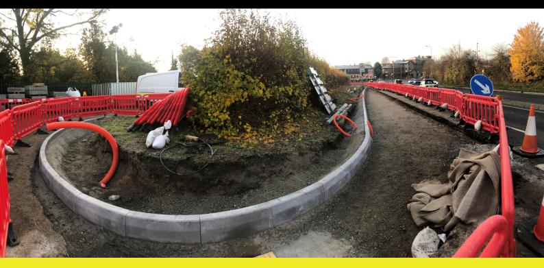
The Channels project saw Henderson & Taylor creating an additional lane to ease traffic flow at the junction of Recotry Road with Chelmer Valley Road. The project involved planing out, embankment stabilisation, drainage, kerbing, utilities management, and surfacing, as well as building a tobermore retaining wall to widen the road without disturbing the adjacent cemetary.
