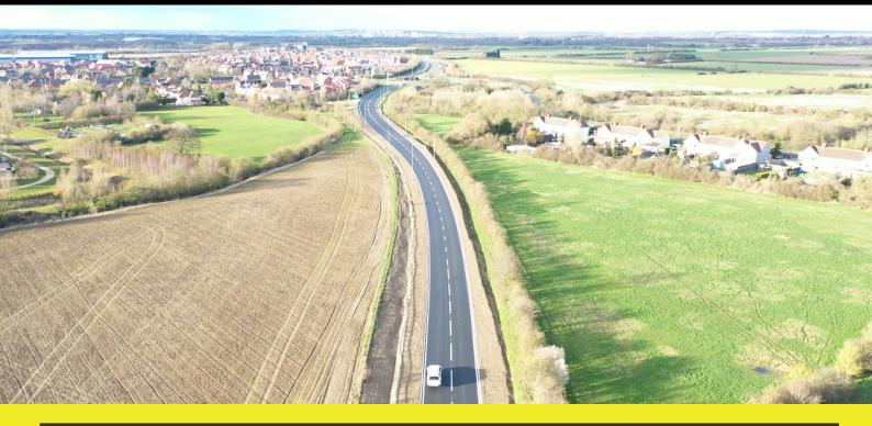
The reconstruction of the A6 Bypass at Wilstead for Bedford Borough Council took place between July 2019 and March 2020 and involved the full removal of the existing failed bypass and rebuilding of the new surface, including extensive drainage works, kerbing, surfacing, fencing, lining, and signage, with all the associated works.
